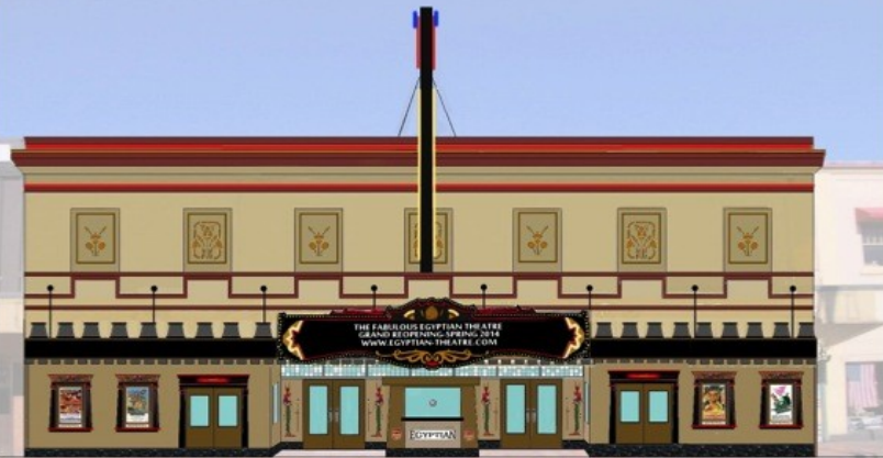
The new façade
